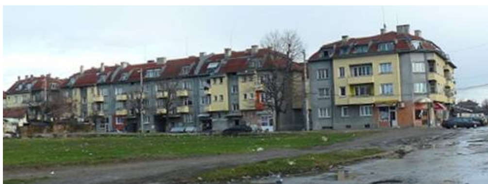
New social housing construction in Hristo Botev neighbourhood in Sofia (BG)
